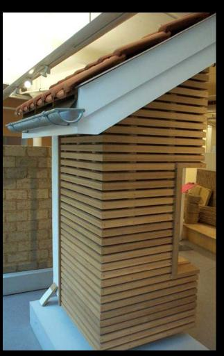
Hygroscopic insulation maintain their performance even when wet Vapour and water released when conditions permit No need for Vapour Barrier VB Use vapour permeable construction 5:1 ratio vr inside:outside **Air Tightness Layer ATL**
