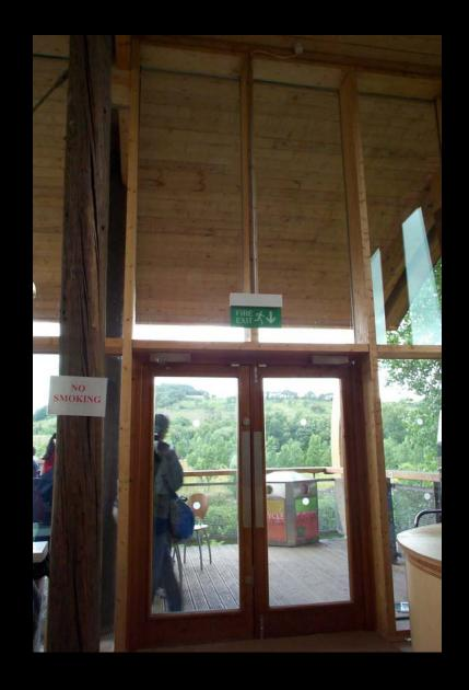
**Timber Structure, Curtain Walling,** Doors and Boarding, Minimise cold bridges Less condensation Natural sustainable material **Mostly recycled** timber
