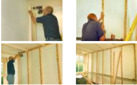
Kitchen - Installing EcoStuds
