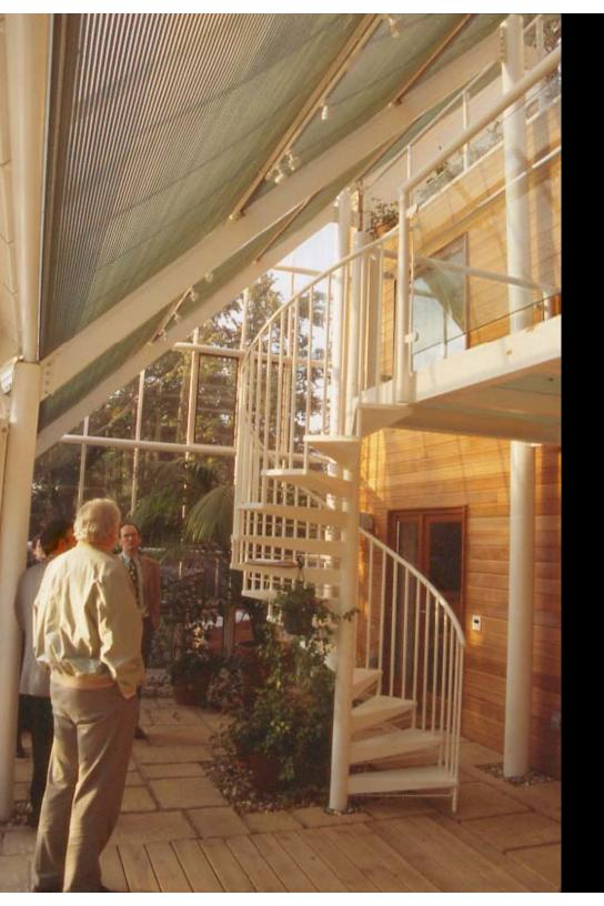
Internal Solar shading No Thermal Mass on rear wall Some thermal mass on floor
