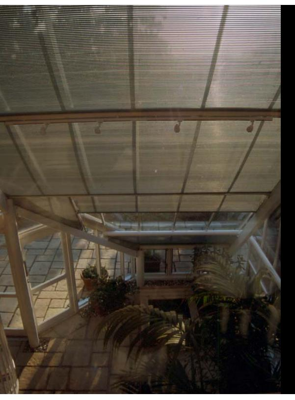
Internal solar shading: catches solar radiation heats up and re-radiates heat inwards. Energy efficient light fittings?
