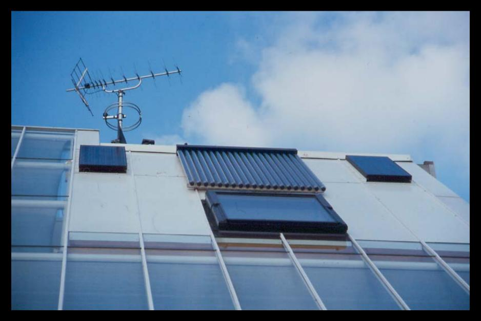
Solar Thermal ET for Hot Water Roof window & minimal PV
