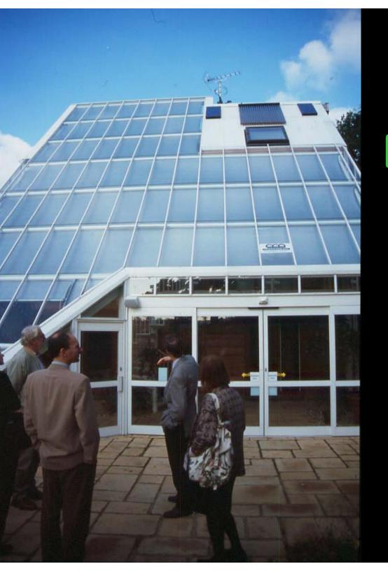
Doors: provide low level ventilation Windows: none at top Internal solar shading: internal radiant heating & thermal stress
