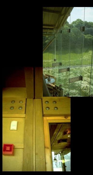
Methods of Assembly Fixings and **Fastenings** permit deconstruction and reuse of structural components
