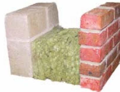
thermal mass and insulation at BedZED
