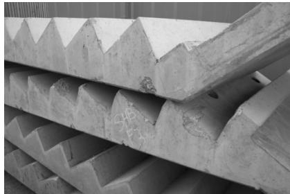
Damage by methods of work 3.2% Specify Cast-in Lifting eyes sockets; require protection, consider repair before condemning
