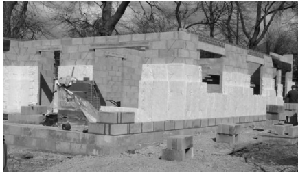
Attempting to reduce waste: creating cold bridges Cold bridge reducing ties won't make up for: brick inner leaf and brick padstones for lintels Omitting jamb returns reduces waste and cold bridges
