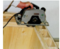
(above) The blocks are easily cut and adapted to most design details.
