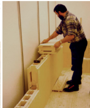
(right) This wall being constructed at an exhibition was very rapidly built using the Steko system.
