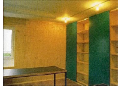
(below) This completed room gives away few clues as to how it was built - and the blocks provide an attractive finish that needs little further treatment.
