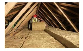
Step 2: roll another layer at 90 degrees to the first layer, to give the total required thickness
