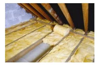
Step 1: lay insulation between the joists (usually 75 or 100mm tall)
