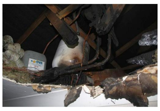
live conductors which caused a fire involving the timbers within the loft space.
