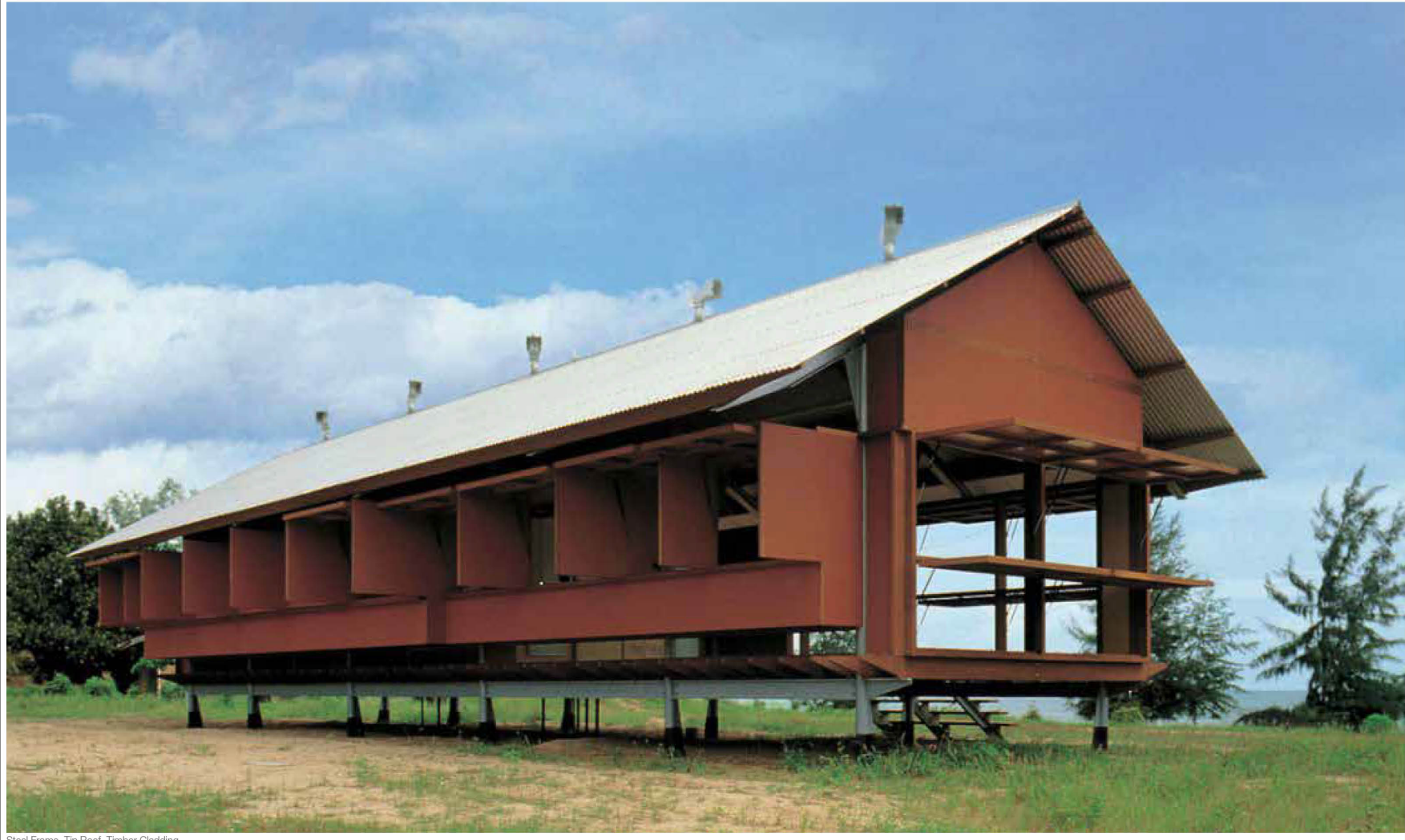
Steel Frame, Tin Roof, Timber Cladding
