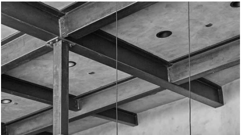
Example Steel Frame carrying Concrete Floor Deck
