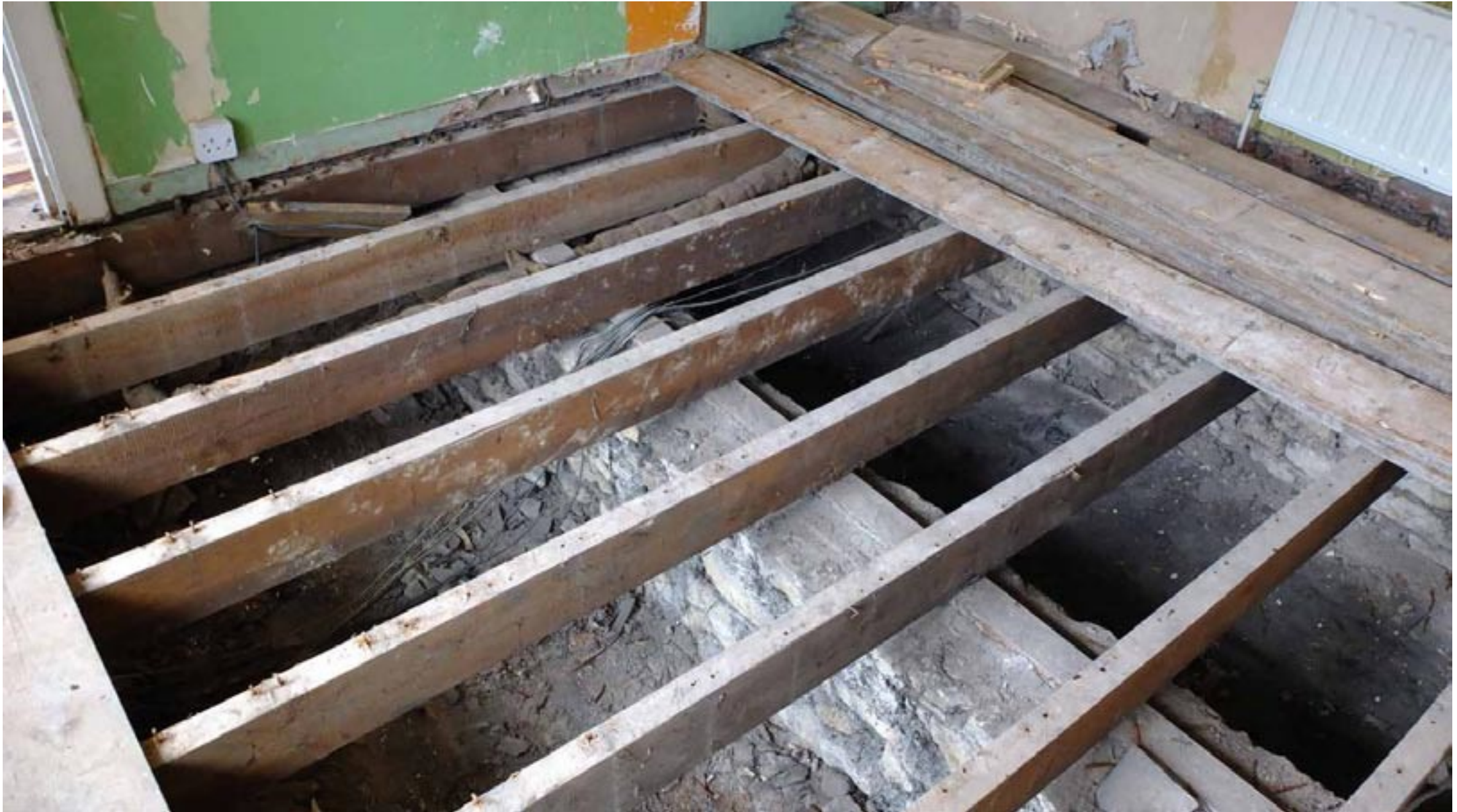
Example suspended timber floor
