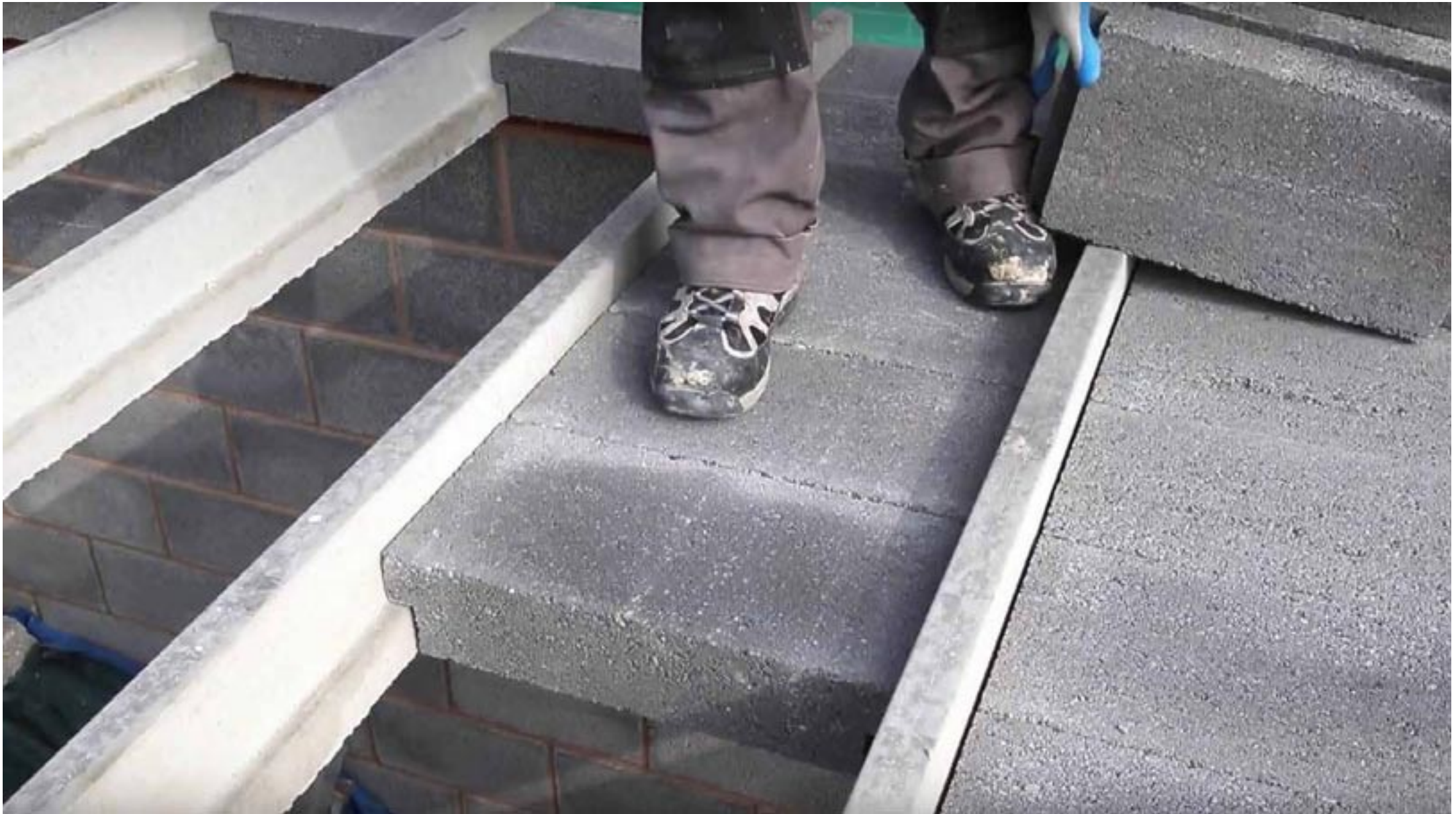
Example suspended concrete floor
