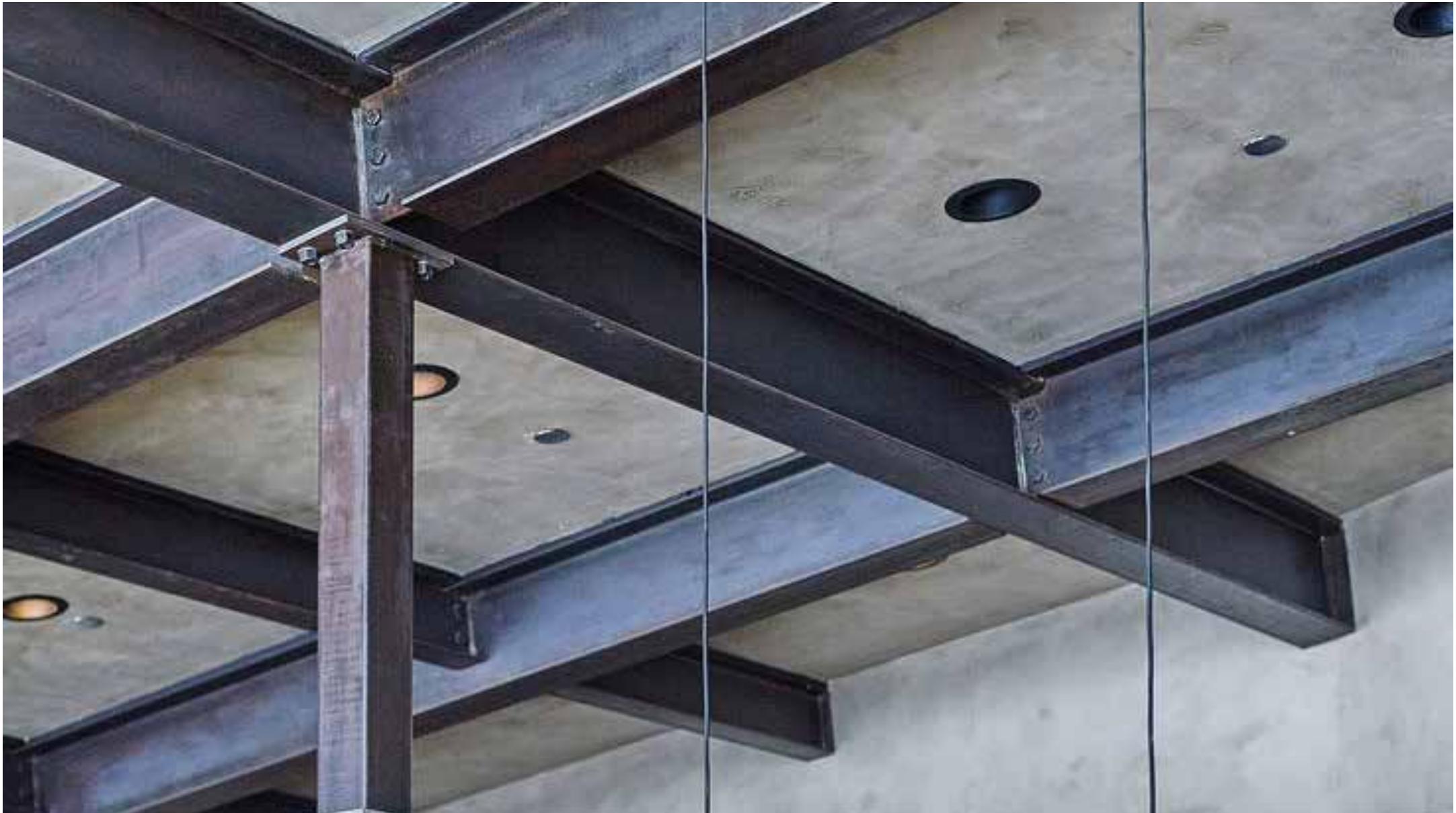
Example Steel Frame carrying Concrete Floor Deck
