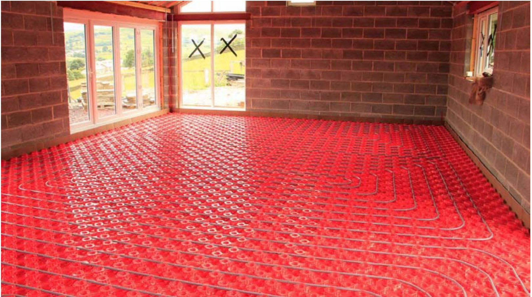
Under Floor Heating Site Photo
