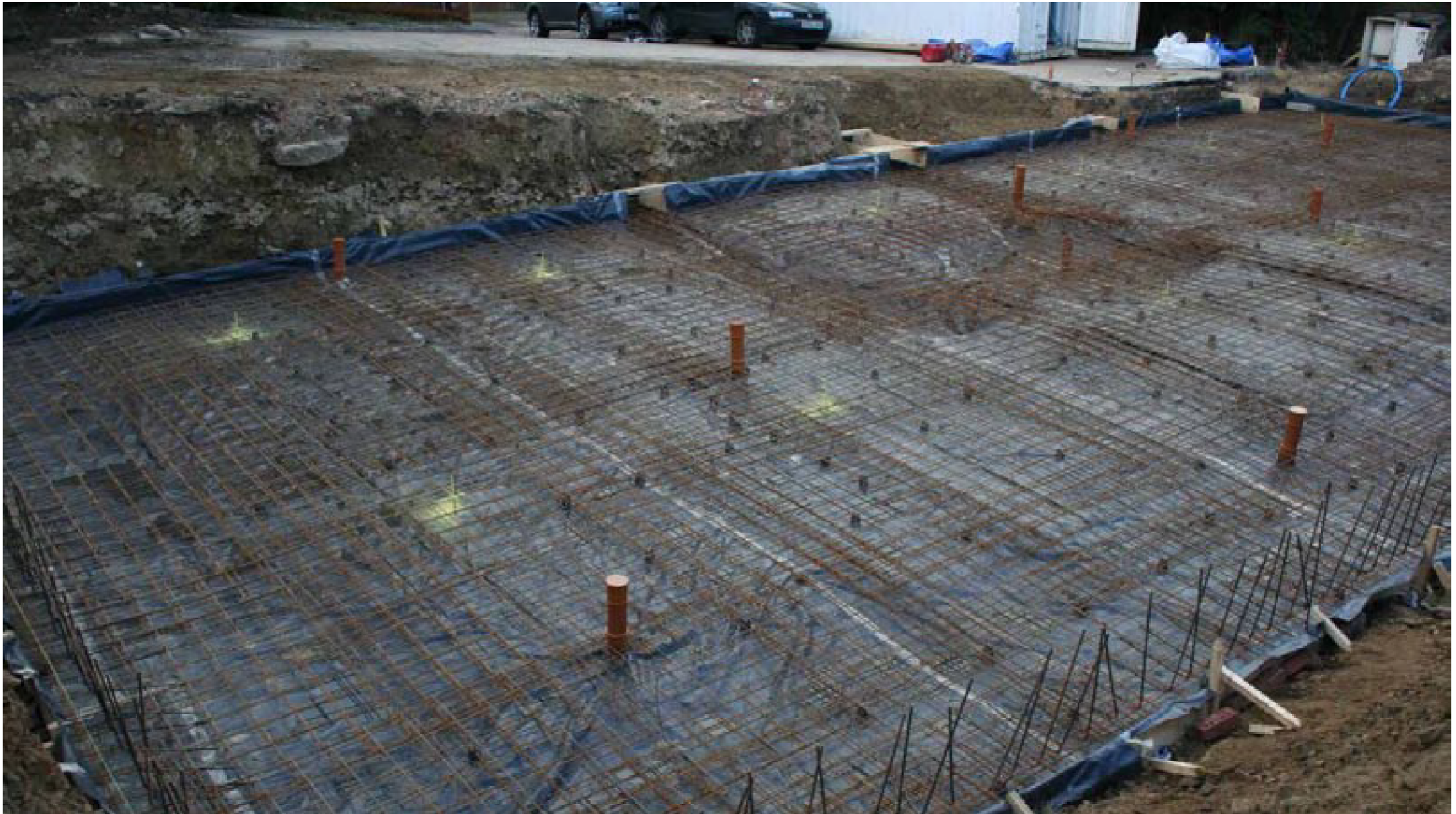
Ground Bearing Floor Site photo
