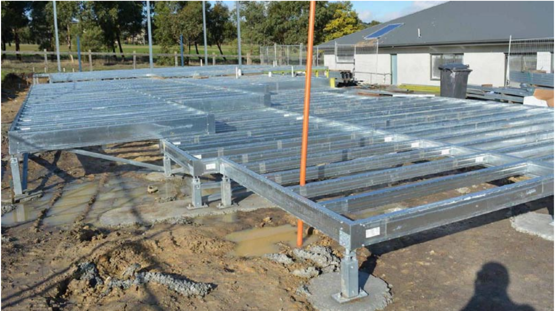
Example suspended steel floor
