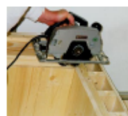
(above) The blocks are easily cut and adapted to most design details.
