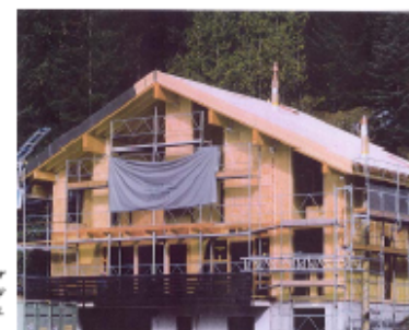
(top right) A building under construction showing 3 storey load bearing Steko walls.
