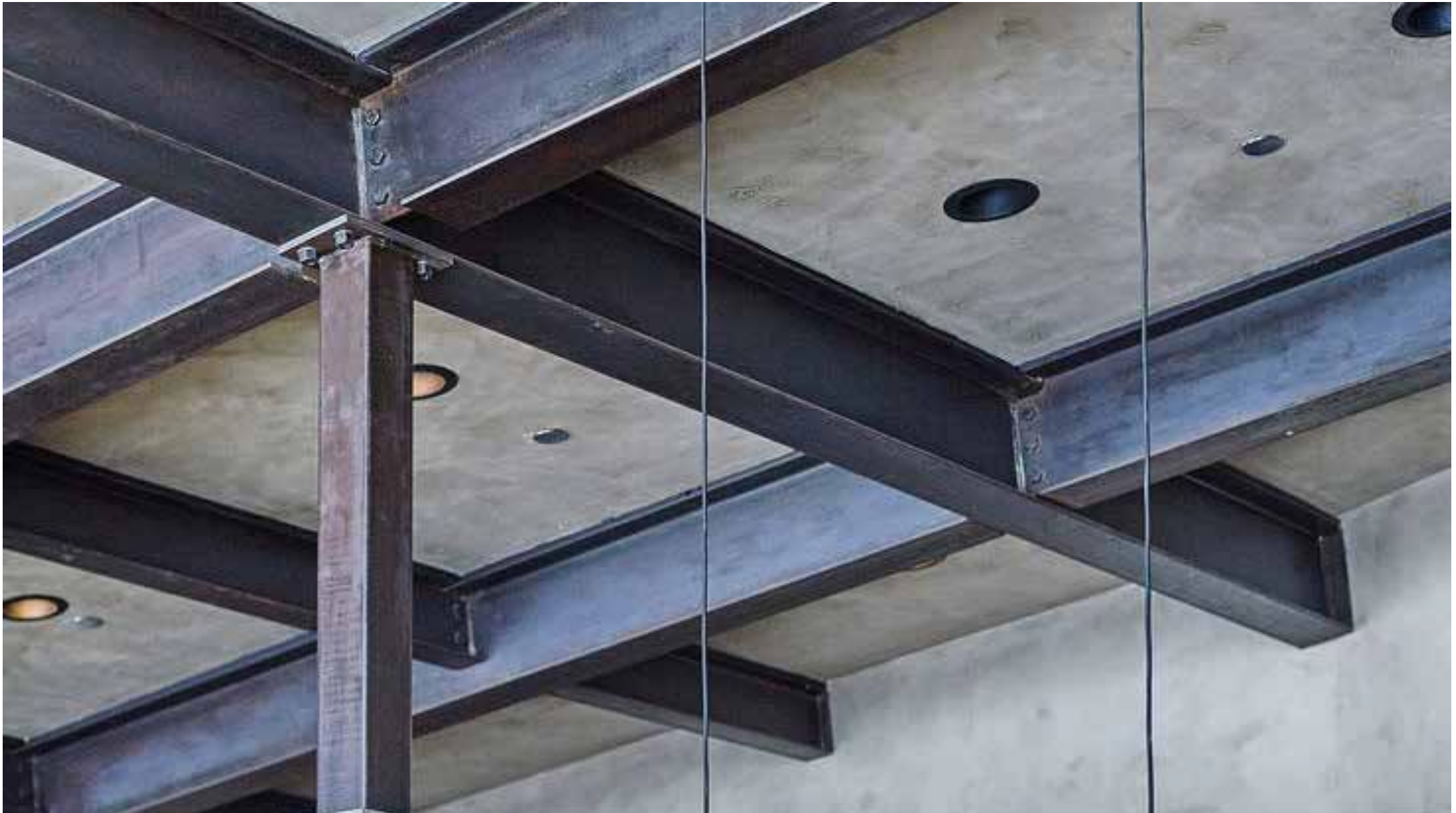
Example Steel Frame carrying Concrete Floor Deck
